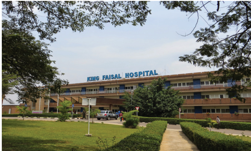
King Faisal Hospital (Source: Google Rwanda Image)
